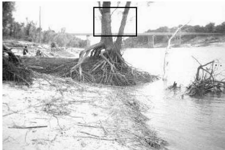
Fig. 7. Trinity River channel just downstream of Livingston Dam. The exposed tree roots are indicative of recent channel scour and bank erosion. The box highlights light-colored stains on the tree, derived from scour of gray clay bed sediments during high flows.
